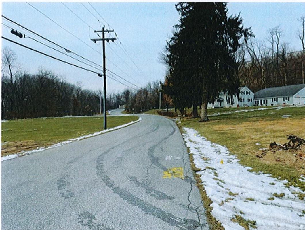
PHOTO 2 - Standing along Church Road at western property line facing North.
